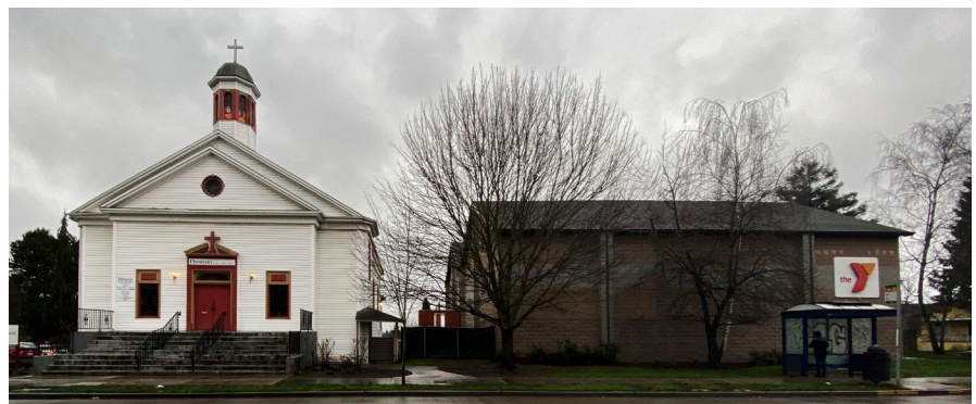
Existing Ebenezer AME Zion Church and Meredith Mathews East Madison YMCA seen from 23rd Ave AUBREE NICHOLS
